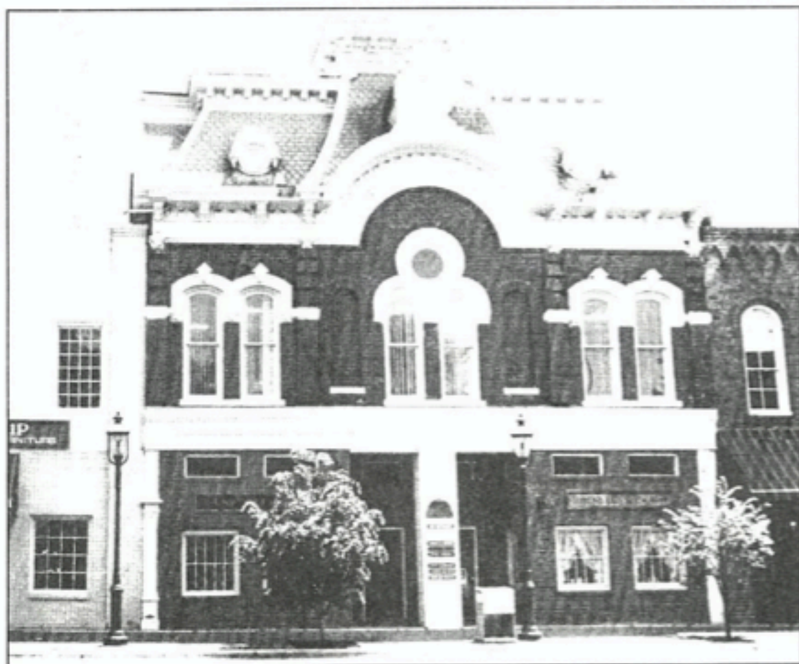
Front view before Allan Jones' restoration. Note the small trees.
